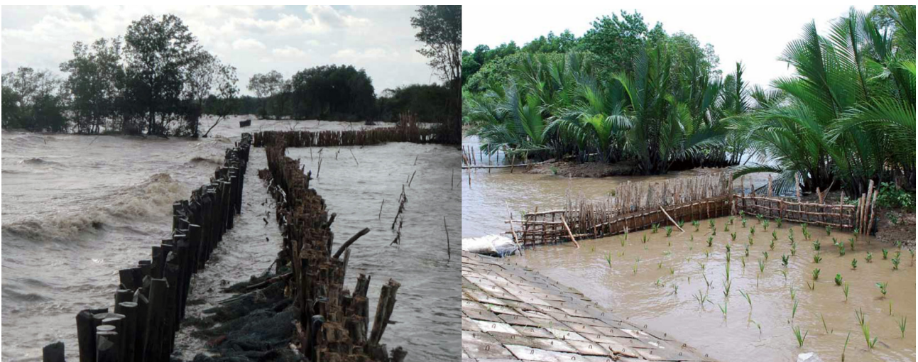
Figure 6-4 Wave break fence for stabilising heavily eroded coastlines and sediment trap fences for areas of low erosion and for natural regeneration used in Vam Ray restoration project
